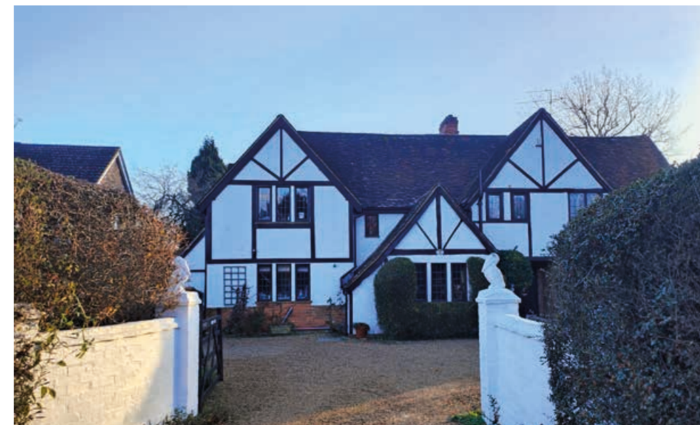
6. Timber framed house, Cox Green Lane
