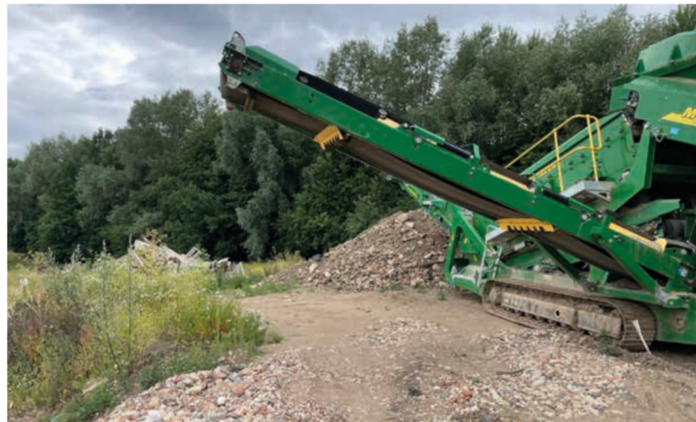
Eastern field used by soil processing and turf business
